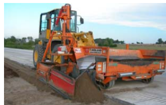
Use of recycled concrete and asphalt in highway construction
